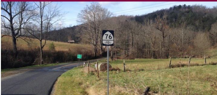
Route 76 at the Montgomery-Roanoke county line.
